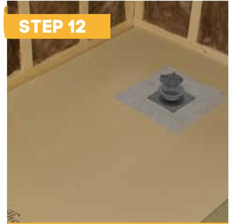
Using the securing tool supplied with the drain, screw the threaded waste collar into the drain body before the adhesive hardens. Care must be taken to fully tighten the assembly to ensure a watertight seal is achieved. The securing tool should be left within the drain body at this stage to protect against debris falling into the drain during tiling and grouting.
