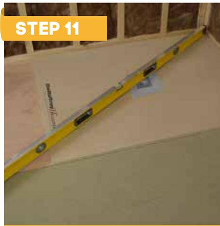
With care place the DeltaTray into the adhesive. Make sure the rubber seal of the drain remains firmly seated on the drain body. Apply moderate pressure to the entire surface of the tray and around the drain aperture, making sure there are no hollow spots beneath the tray.
