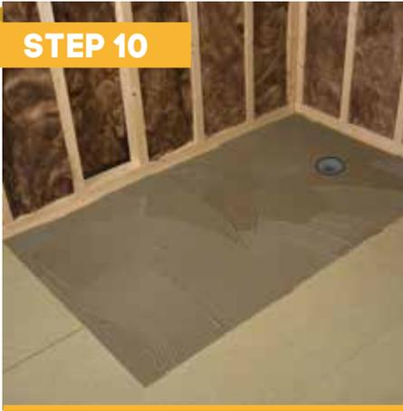
With the installation of the supporting platform fully prepared and all checks complete, the DeltaTray can now be fixed into place. DeltaTray is permanently fixed in place using a good quality, cement based rapid setting flexible tile adhesive. Apply the adhesive with a thick bed notched trowel to the area where the DeltaTray is to be placed.
