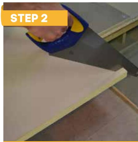
If the drain conflicts with a joist or other obstruction, the tray sides can be trimmed to alter the drain position. Refer to trimming your DeltaTray for details.
