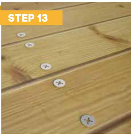
With the DeltaTray fixed into the adhesive, the surrounding floor area can now be overlaid with DeltaBoard. It is very important that the existing floorboard/chipboard must be securely fastened to the joists using suitable screws. If previously fixed with nails, additional screws should still be used.
