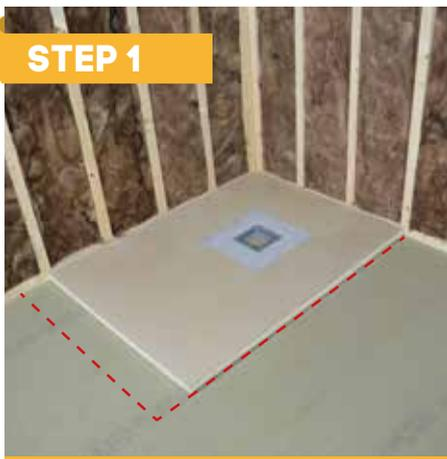
Clear the working area from loose debris and grease. Place DeltaTray onto floorboard/ chipboard to allow marking out of the tray perimeter onto the floor. When setting out the position of the tray it is important to remove the floorboard/chipboard past the edge of the tray and back to the centre of the next joist. Check that the position of the drain does not conflict with joists below the floorboard/ chipboard.
