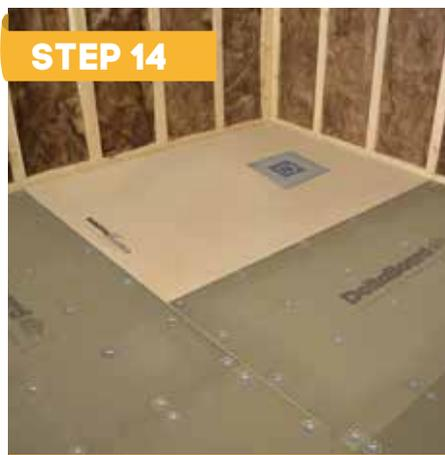
If the DeltaBoard is to be installed using a dry fix method, PCS washers should be positioned at approx. 200mm centres. It is important to use the correct length of screw to avoid penetration of the floorboard/chipboard when fixing the DeltaBoard in place.
