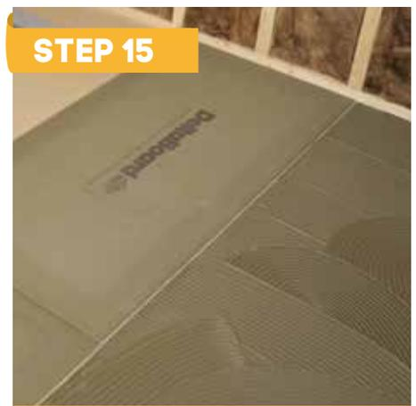
If using a cement based adhesive to fix the DeltaBoard, the existing floor surface must be primed with a suitable floor primer (refer to adhesive packaging for instruction.) Apply a solid bed of adhesive using a thick bed notched trowel and firm down the DeltaBoard into the adhesive bed.
